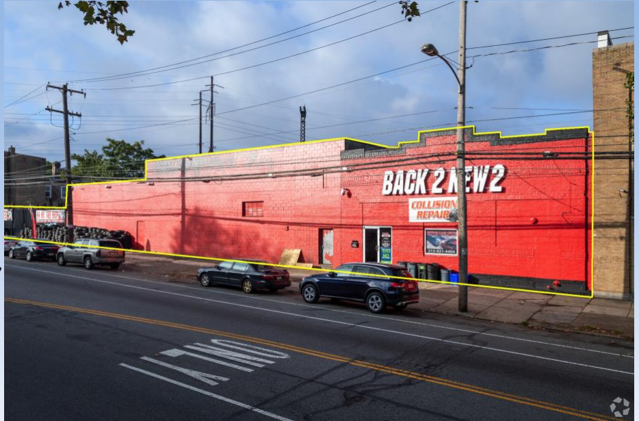
Rear Entry & Yard Lex Street
